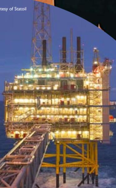
Carbon capture and storage is feasible. Carbon dioxide extracted from gas production on Statoil's Sleipner West field in the Norwegian North Sea is stored 1,000 metres below ground instead of being released to the air. The process, in use since 1996, sequesters about 2,800 tonnes of CO<sub>2</sub> every day.
