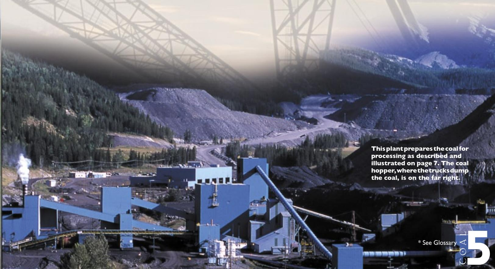
This plant prepares the coal for processing as described and illustrated on page 7. The coal hopper, where the trucks dump the coal, is on the far right.
